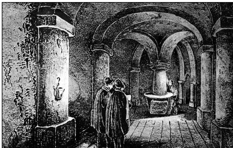
Fot. 3. Komora Schuckmana Phot. 3. Schuckman's chamber
