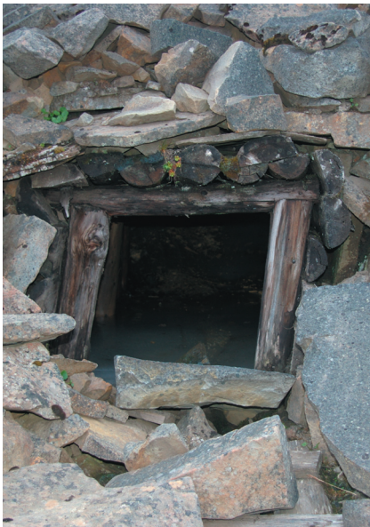
Ryc. 6. Wlot sztolni G2b–δ Fig. 6. Entrance of adit no. G2b–δ
